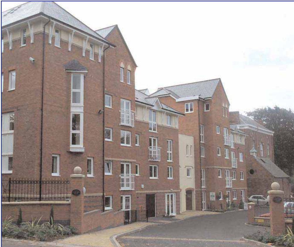
This development has used the steep topography of the site to its advantage whilst also respecting the scale, style and materials of the adjacent Victorian villa.
