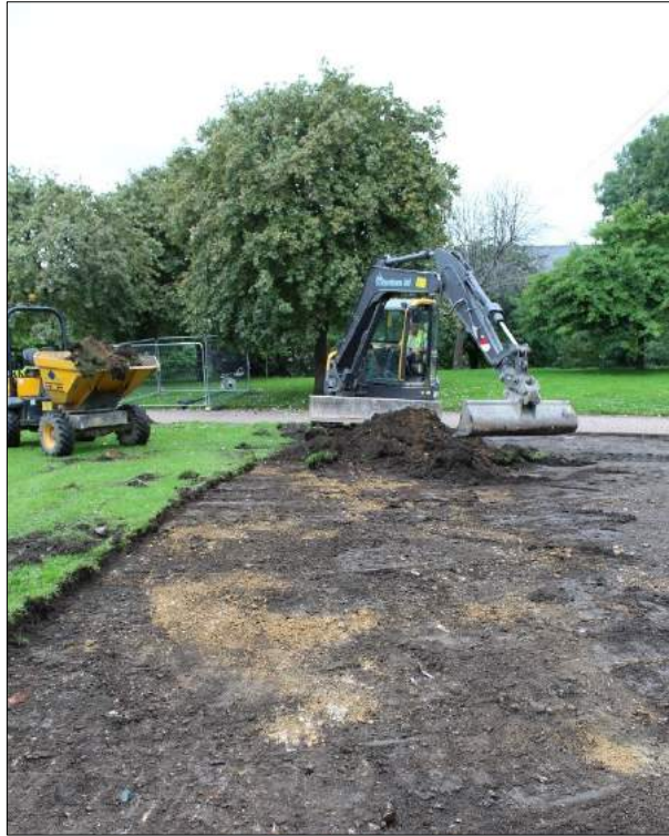
Plate 9: Topsoil stripping of area of the compound, looking west
