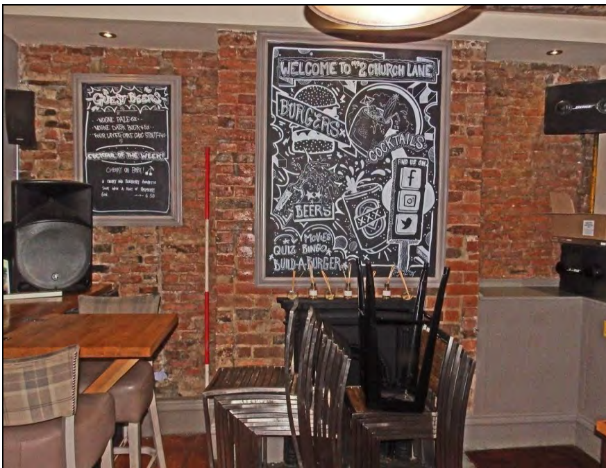
Illus. 15: Wall E, with blocked doorway to left of chimney breast
