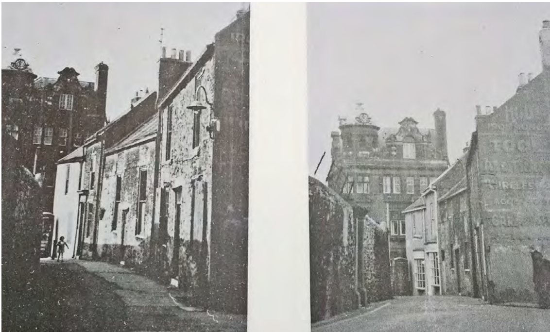
Illus. 08i & ii: The west side of the buildings on Church Lane before and after alterations in the 1970s.
