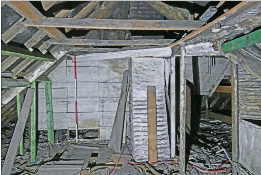
Illus. 20: Attic of the Northern Building, west part looking north, showing the lobby on the right linking to the south part of attic, and the partition formed by old broad boards
