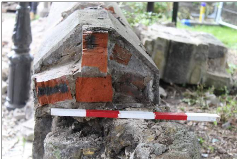
Plate 11: Construction of wall coping, walls 110 and 133, 0.50m scale
