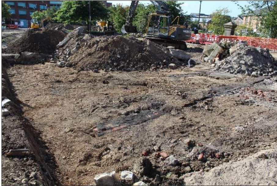
Plate 18: Proposed amphitheatre area during stripping, looking southwest
