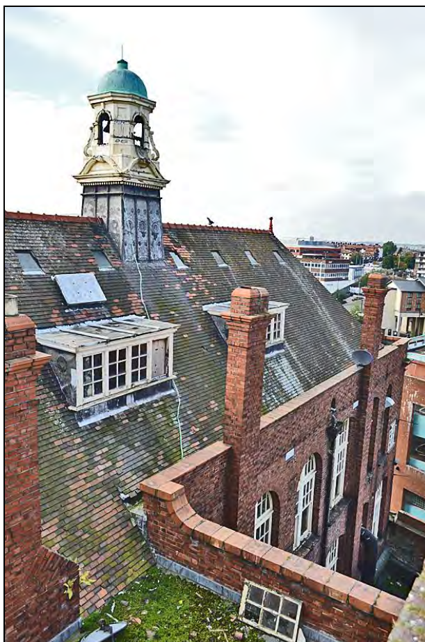
Frontispiece: View from roof level looking north-west towards the north part of the east elevation.
