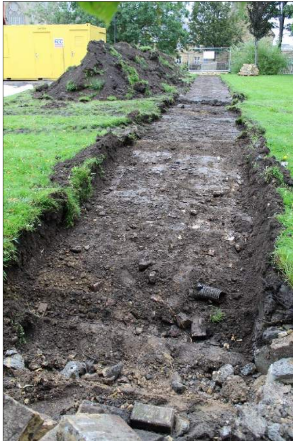
Plate 10: Stripping for temporary footpath, looking north
