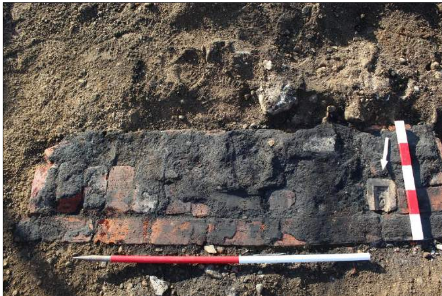
Plate 19: Section of wall foundation 118 showing broken firebrick (arrowed), facing south, 1m and 0.5m scales
