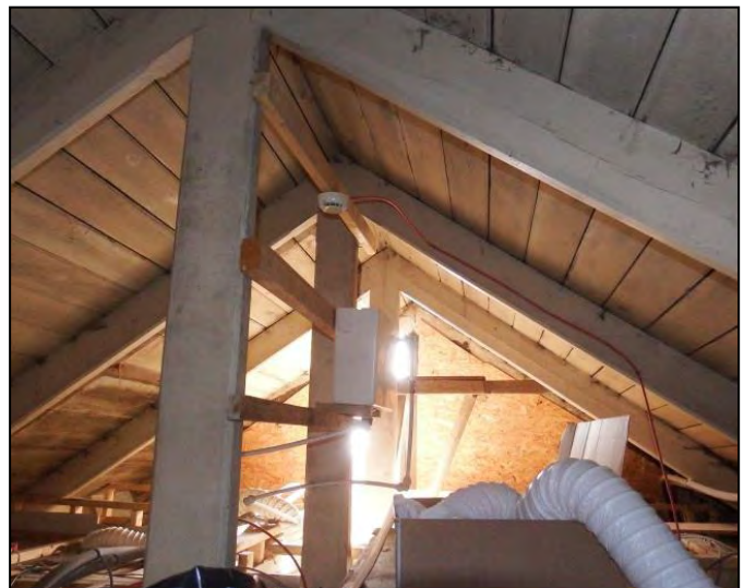
Illus. 22: Rear block roof looking south
