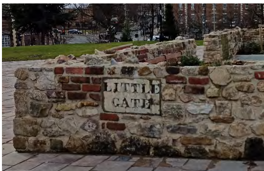
Figure 4.52: Salvaged brick and Concretionary Limestone being used in the new Town Green development
