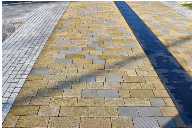
Figure 4.51: White Granite (left) Carboniferous gritstone (buff) Pennant Sandstone (grey) and the Keel row in dark gabbro
