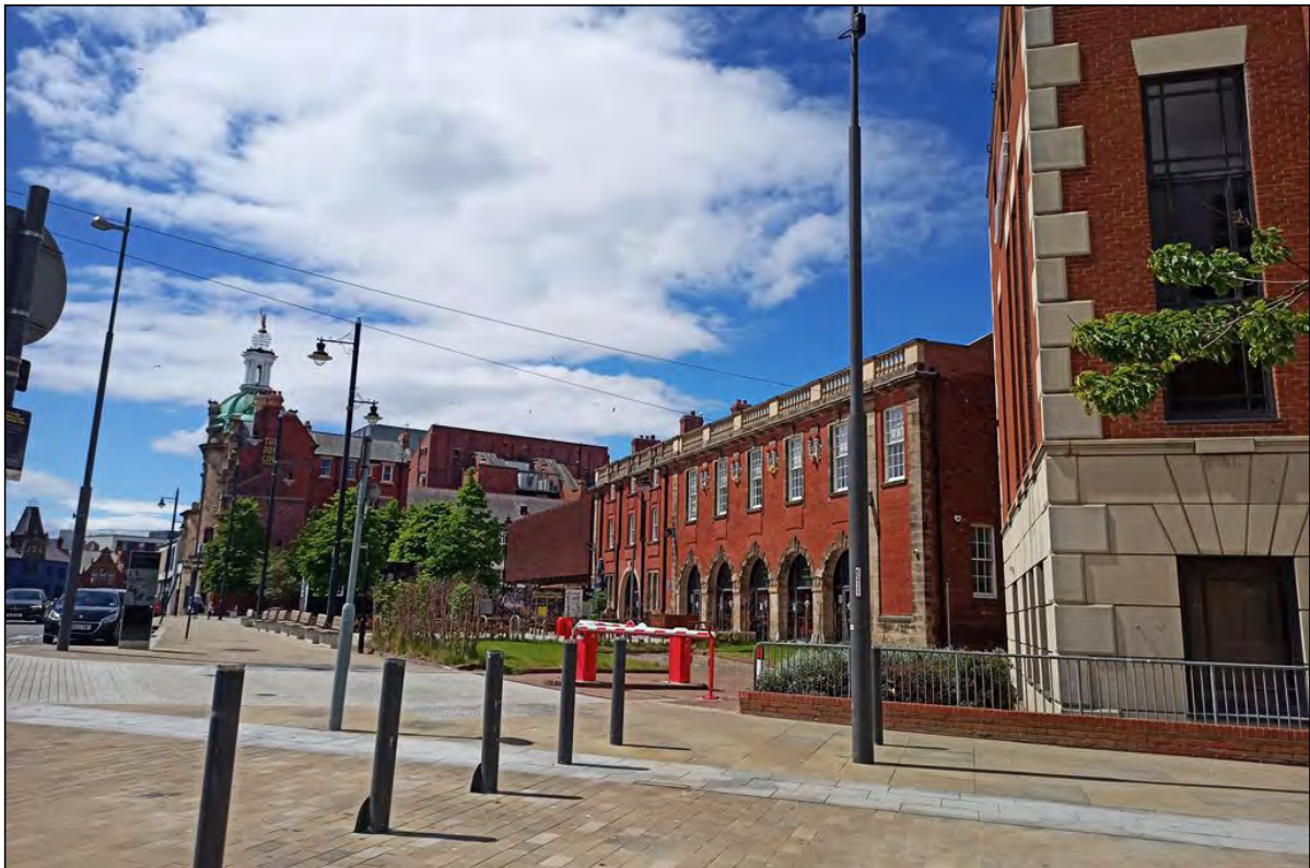
A 2021 view looking westward along High Street West from a similar vantage point today. Demolition of most of the structures in the upper photograph has opened up views of the Fire Station, now adapted as a restaurant/café bar, arts centre and performance space.
