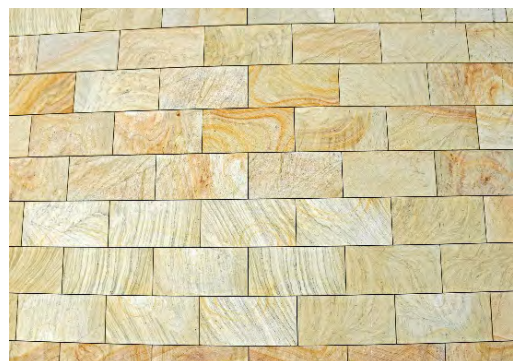
Figure 4.49: Bedding and diagenetic iron patterns in sandstone cladding on the Exchange building
