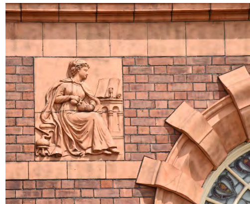
Figure 4.46: Detail of ceramic work on the Galen Building
