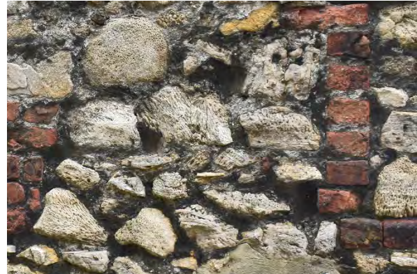
Figure 4.28: Concretionary limestone and brick in the wall by the footpath to Chester Road
