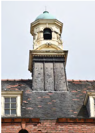
Figure 4.22: Copper and leadwork on the roof of the Galen Building
