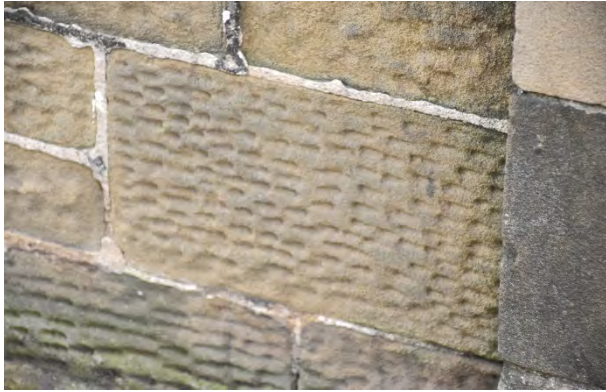
Figure 4.27: Tool markings on cut stone in the boundary wall of the Minster
