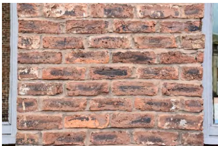
Figure 4.38: Hand cut bricks in Green Terrace
