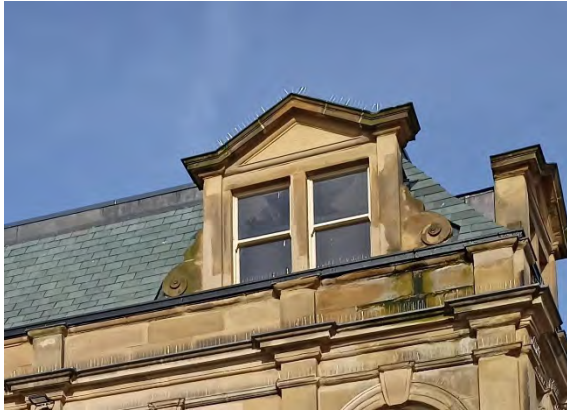
Figure 4.31: Slate roof on the Londonderry Hotel
