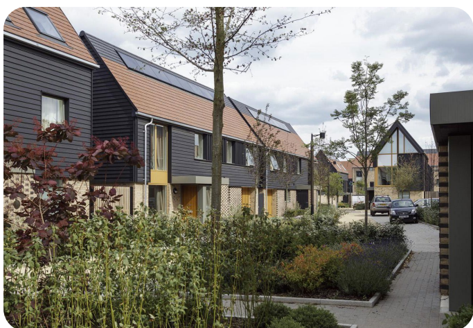
Landscaping: Integrated within streetscene (Abode, Cambridge)
