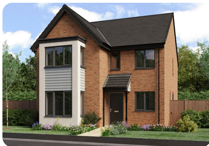
Locally distinctive: Standard house type altered to reflect location (Potters Hill, Sunderland)
