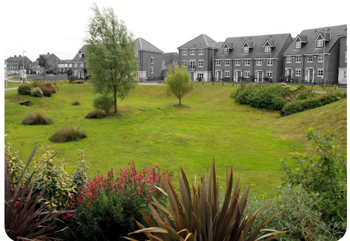
SUDS. Detention basin (susdrain)
