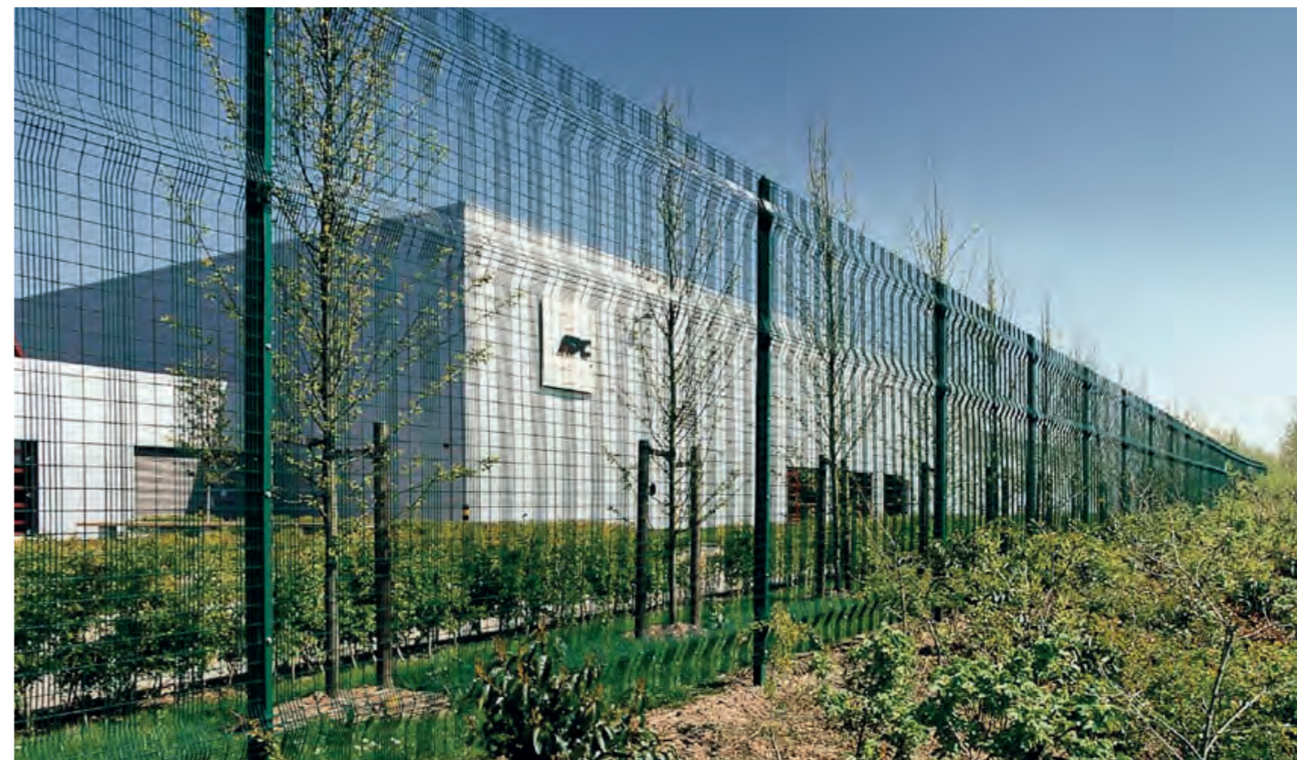
Precedent Wire Mesh Fence, height 2.4m. (RAL 6005, Green)
