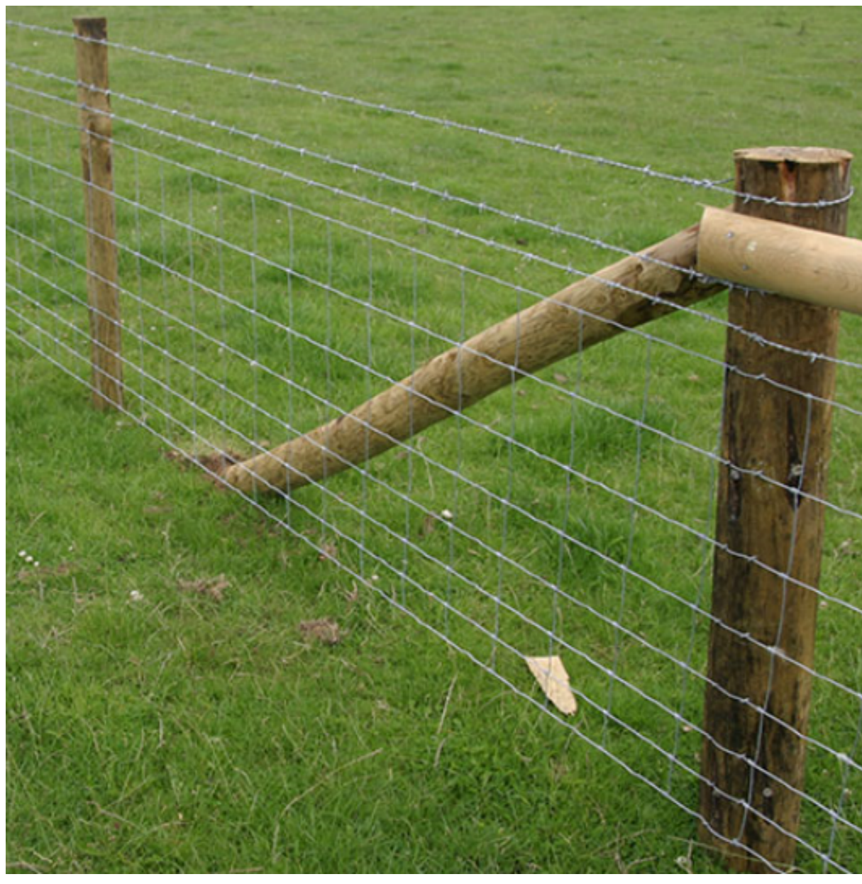
Timber Post and Wire Mesh Fencing 1.2m high
