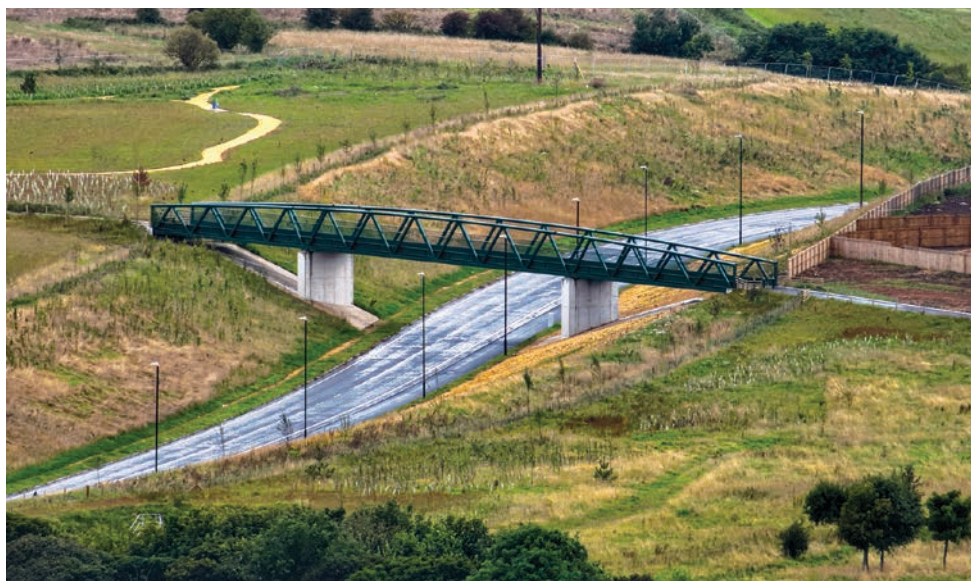
RDLR Non-Motorised User bridge, September 2023
