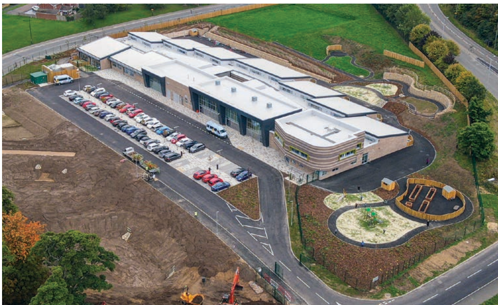
Sunningdale School under construction
